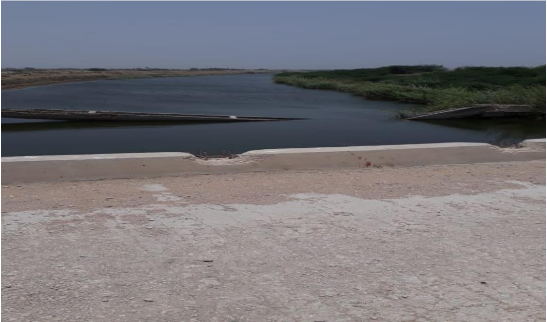
RD 760+600 Water Course
