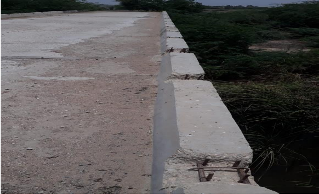
RD 760+600 Village Road Bridge
