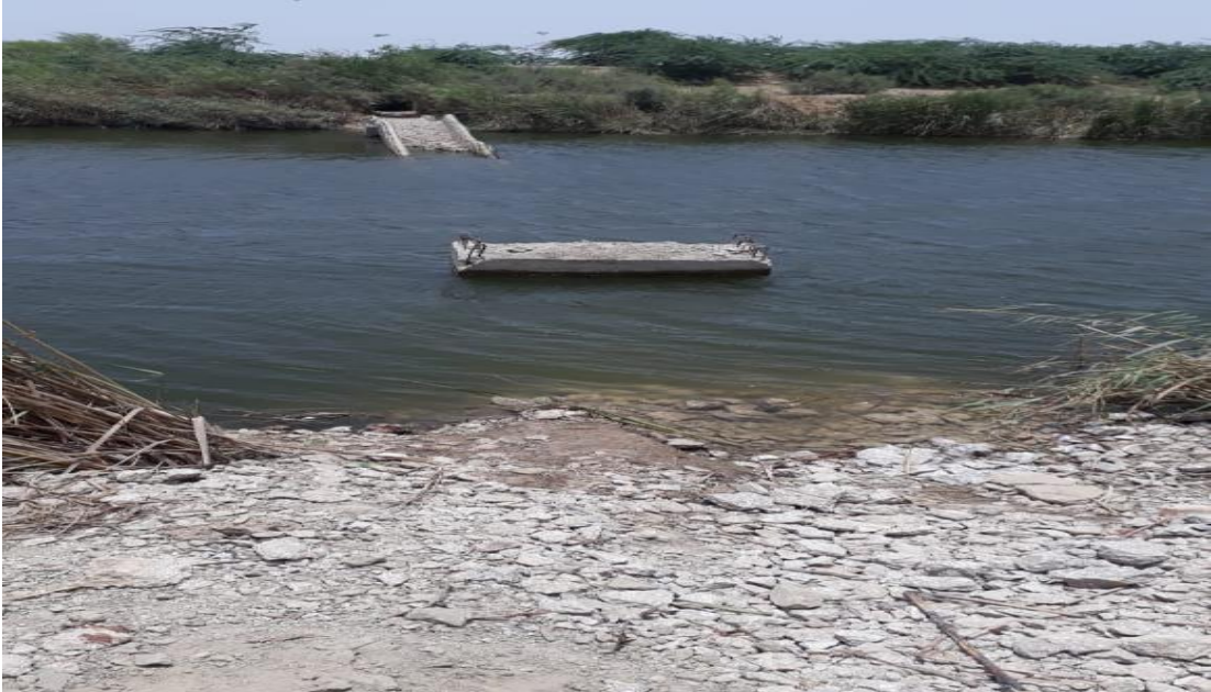
RD 768 Water Course
